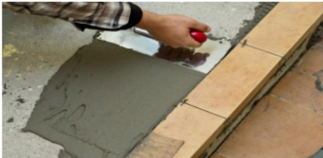
Apply Adhesive using Plain Side of Trowel
