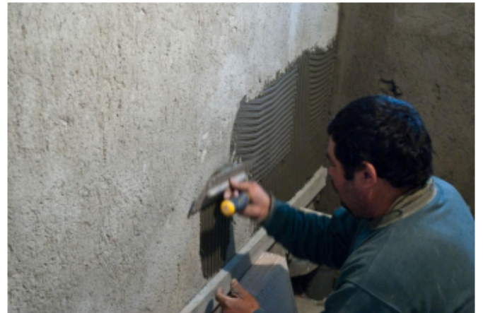
Application of BS Tileasy-F on Wall over smooth levelled / plastered surface.
